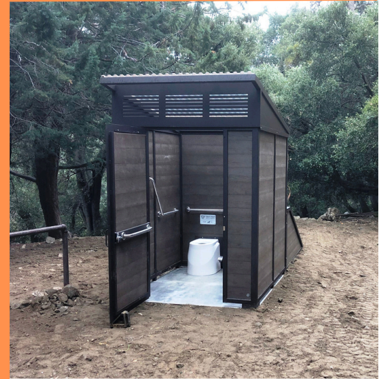
A peek inside the Mt. Lowe ADA building
